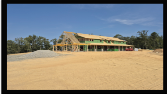
Dry wall and roof are up!
