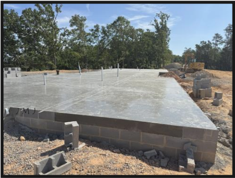
Foundation is ready!
