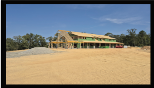
Dry wall and roof are up!
